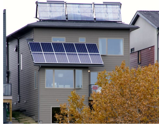
Solar thermal heating and solar photovoltaic panels. Photo credit: David Dodge, GreenEnergyFutures.ca
